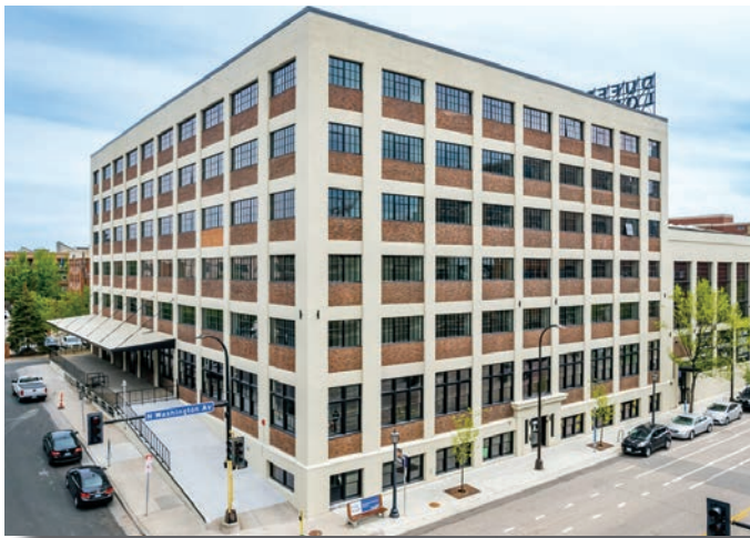
THE DUFFEY LOFTS (FORMERLY C.J. DUFFEY PAPER CO.) Minneapolis, MN Built: 1923
