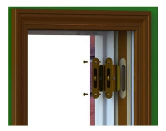
Lower the top sash and cut the balance cords. Remove the top sash and dispose of it properly. Remove the balance chord pulleys. Remove any remaining jamb liner material (if applicable). Insulate the weight pockets and any openings or voids.
