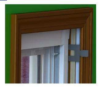
Place a shim at each of the pilot hole locations, and insert a screw into one top corner to hold window in place. Remove sash stop at head of window and replace when screws are tightened. Note: When installing all installation screws make sure to tighten screw so the screw head is flush or slightly dimpled in so screw doesn't interfere with balance shoe.
