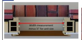
Note: Take measurements at three locations (head, middle, sill for width and left, center, right for height). Use the smallest of the three measurements to ensure the unit can be installed square, level, and plumb.
